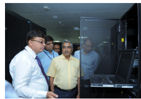
Secretary (Power) & JS evincing keen interest at GUVNL Data Center
